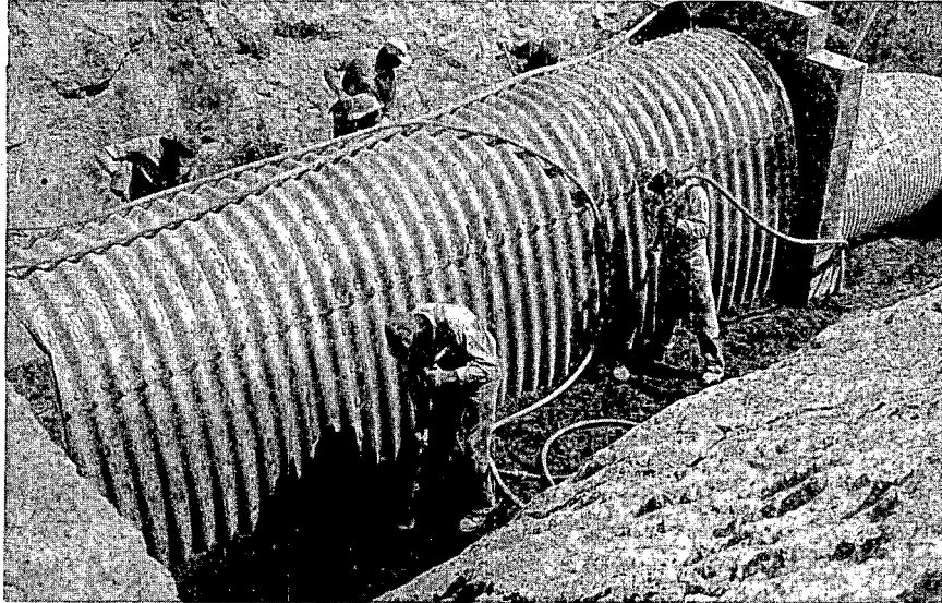
Figure A.7 Tamping backfill with pneumatic tamper.
